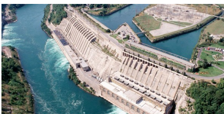
Sir Adam Beck Generating Complex in Niagara Falls, Ontario, the largest source of hydroelectric power in the province.
